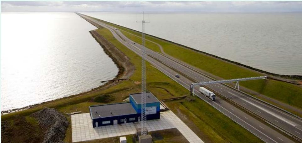
*Thermal energy from surface water: Blue Energy on the Afsluitdijk. In this trial installation, energy is extracted from the difference in salt concentration between freshwater and seawater.*
