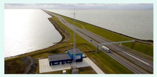
$Thermal\ energy\ from\ surface\ water:\ Blue\ Energy\ on\ the\ Afsluit dijk.\ In\ this\ trial\ installation,\ energy\ is$  $extracted\ from\ the\ difference\ in\ salt\ concentration\ between\ freshwater\ and\ seawater.$
