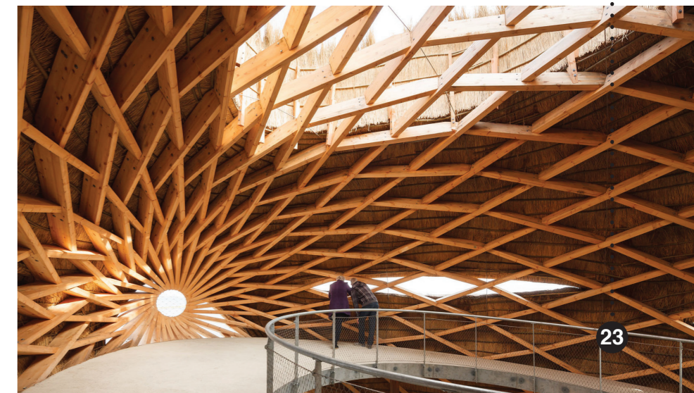
Afb. 3.3 Tijl Observatorium Stellendam. Architect: RAU ism Ro&Ad Bron: RAU
